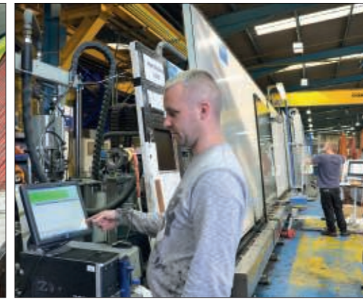
A+W Production Monitor at the discharge from the Bystronic IG-line: each pane produced is registered; in case of breakage or poor units, re-working is initiated.
