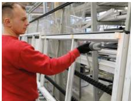
After the employee in glazing has scanned the barcode label on the sash, the A+W Cantor system automatically provides the sheet in question from the glass buffer
